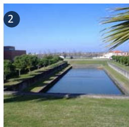
UA – Retention basin
